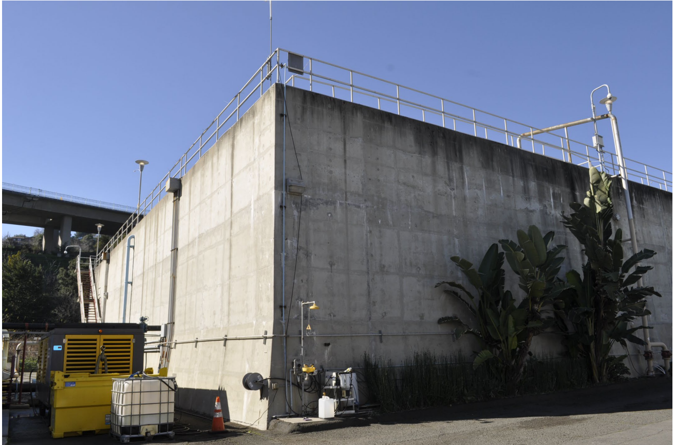
Photograph 9. A portion of the sewage treatment structure at the Philip F. Meads Water Treatment Facility operated by C& H Sugar Company.
