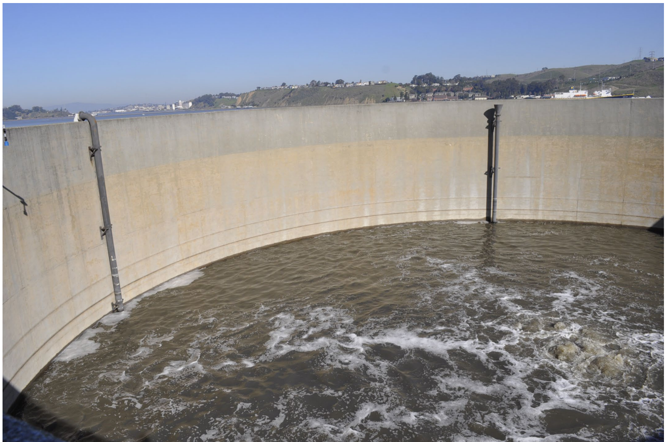
Photograph 6. The interior of the tank. From a distance, the concrete surface showed no distress.
