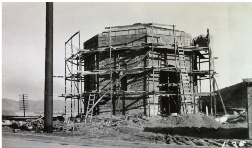
Figure 6: Memorial Hall under construction circa 1924. Note the scored plaster is being applied. Photo from the collection of the Crockett Museum and Historical Society.
