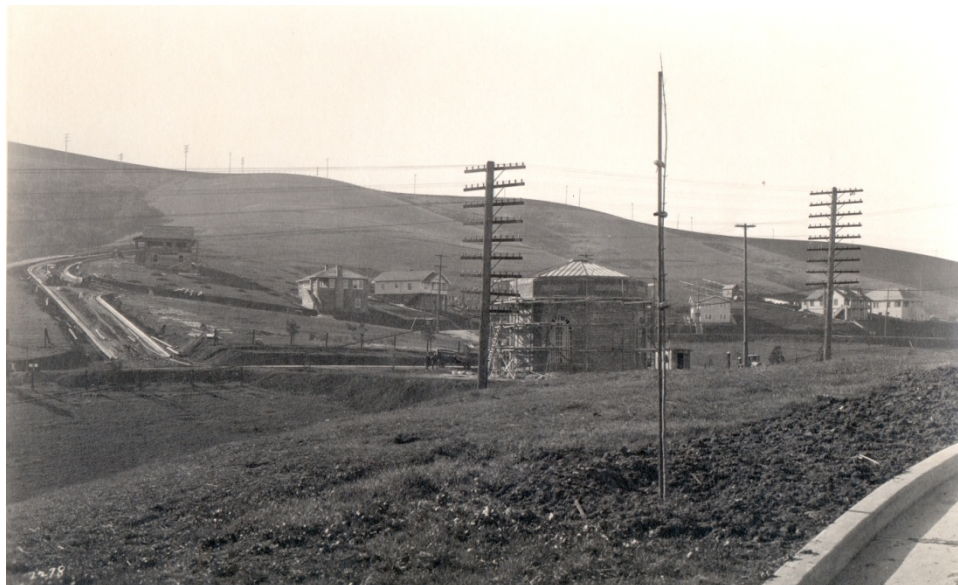
Figure 5: Memorial Hall under construction, looking southwest, circa 1924. Photo from the collection of the Crockett Museum and Historical Society.
