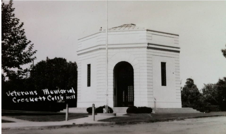
Figure 9: Postcard of Memorial Hall after the 1938 basement reconstruction and re-landscaping. Note only three concrete steps and a base are visible.
