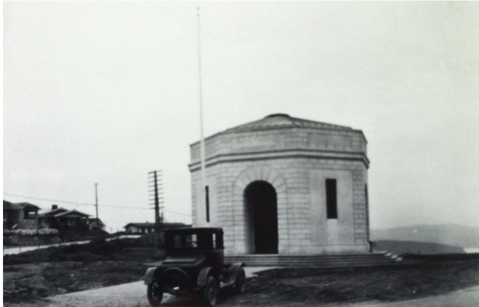
Figure 7: Memorial Hall just completed, looking northeast, circa 1924-25. Note there is no landscaping and there are four concrete steps and a base visible at the plinth. Photo from the collection of the Crockett Museum and Historical Society.
